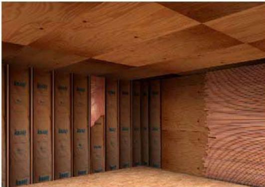
A decorative option to cover your walls and ceiling would be to apply tongue and groove material that complements the wood, stain, and/or lacquer that will be on your racking. You will first need to screw 3/4" marine grade plywood on your walls and ceiling so that you will be able to attach your tongue and groove.
