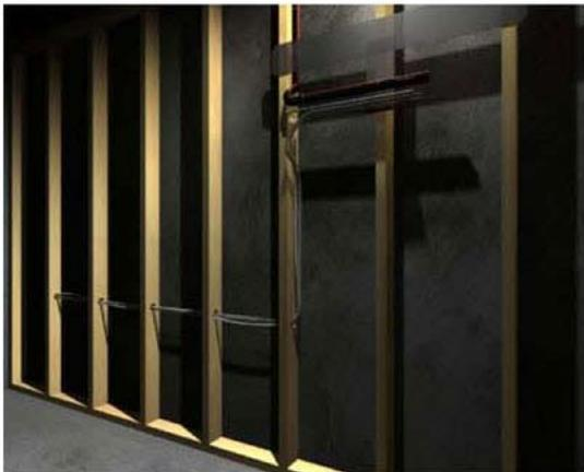
If you are purchasing a WineZone ductless split you will need to run the line set at this stage. The line set is run from the ductless split location to the condenser location, standard condensers are located outdoors, but indoor option is available. You will also need to run a drain line and electric at this time. NOTE: The mounting plate shown is for clarity and is not installed until unit is on site and cellar wall is complete.
