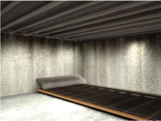
If this is new construction and you are not going to use spray foam, then it is recommended that you install a 6 mil vapor barrier on the back side of your wall studs before lifting them into position. You will also need to wrap your ceiling joists as shown. In some areas the local code specifies all vapor barriers must be installed on the warm side of the cellar. In those areas we highly recommend you switch to the spray foam insulation.
