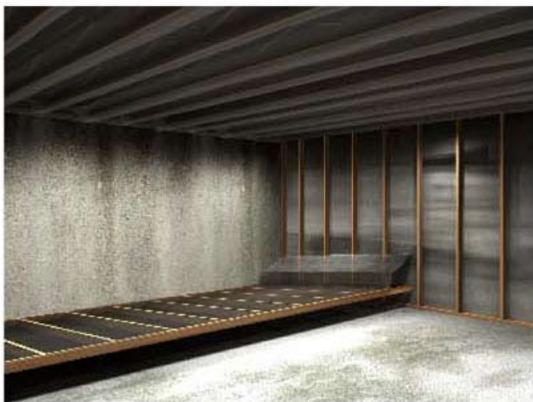
Make sure to leave excess vapor barrier at the corners so that you can wrap it, overlap the seams and tuck tape (not duct tape) them shut. Then fill all holes in studs and joists with fire rated penetration sealant to reduce air movement.
